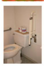
Another simpler, safety item was installed in the handicap washroom - a drop-down support bar. This bar is attached to the back wall and will give people who need it stability on both sides of the toilet.
